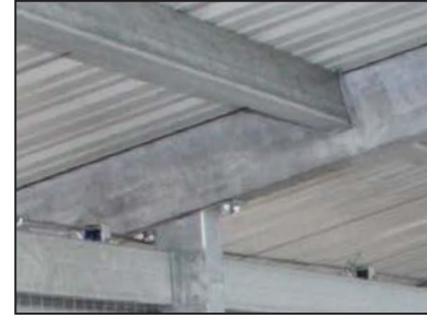
Purlin Design Eliminates Bird Roost
